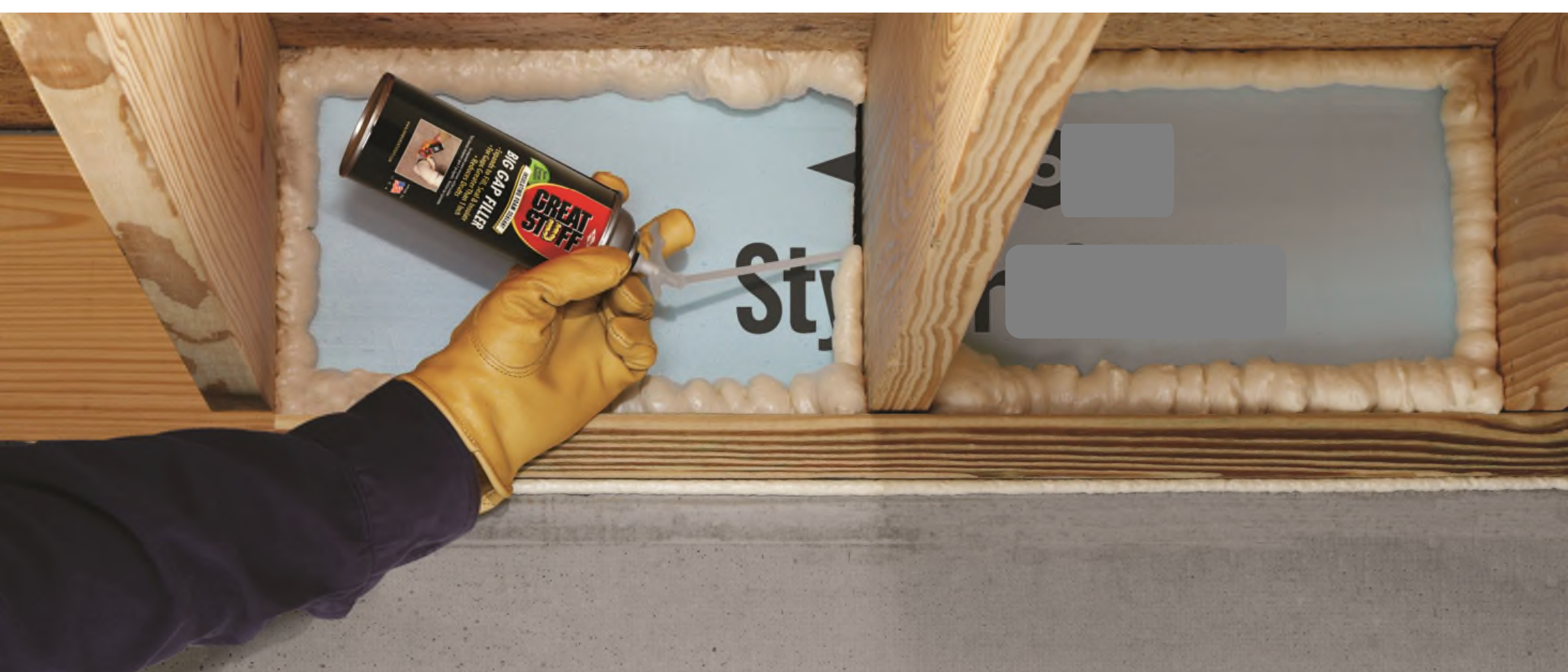
Rim Joist pic of Rigid foam picture framed
